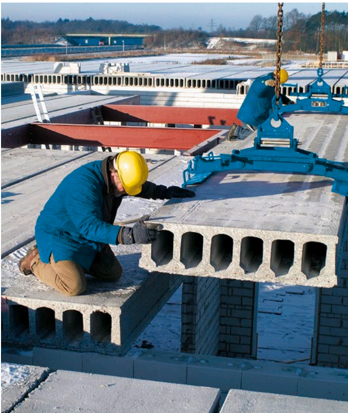
The hollow-core slabs are cut to size and shipped to construction sites with pre-cut openings for plumbing and electrical lines.
